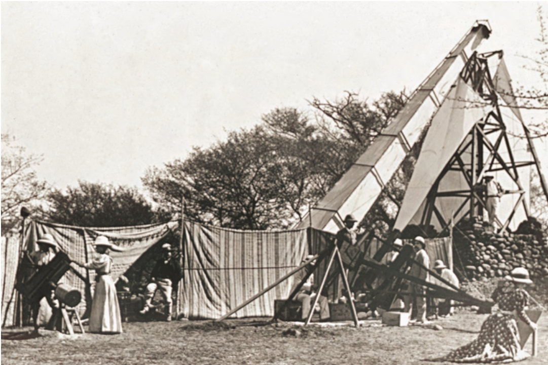
The 40 ft-long telescope of California's Lick Observatory set up near Bombay at Jeur, India to observe the total eclipse of the Sun on January 22, 1898. The cumbersome, long-focus telescope used a 5-inch lens to project an image of the Moon 4 inches in diameter and the corona up to 10 inches across, on 18 x 22 inch glass photographic plates. A series of these were adroitly inserted and removed from the focal plane by hand, one at a time, in the dark of the eclipsed Sun, at this site within a deep pit dug beneath the striped tent. The telescope, called "Jumbo," was taken to fifteen total solar eclipses on six continents from 1893 through 1932, each affording an opportunity of but a few minutes to see the fleeting corona of the Sun.
